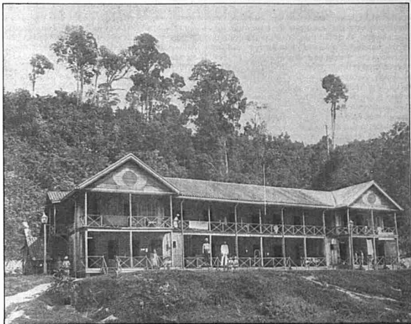
BARRACKS AT SANDAKAN, THE CAPITAL OF BRITISH NORTH BORNEO
